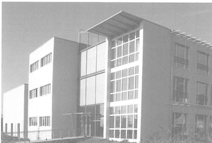
Production and office building in Zwingenberg, Germany Photo: Passive House Institute
