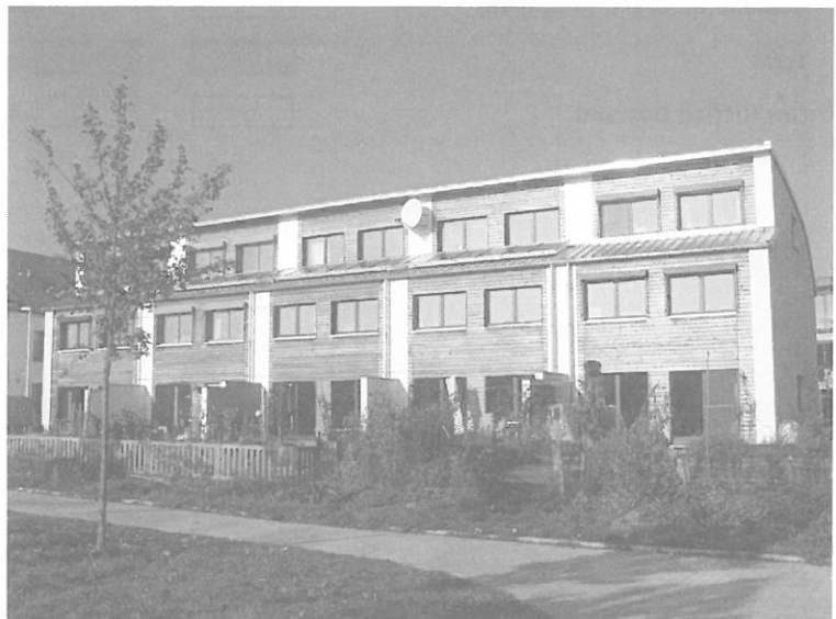
5 Terraced houses in Aachen, Germany Photo: Linie4 Architekten
