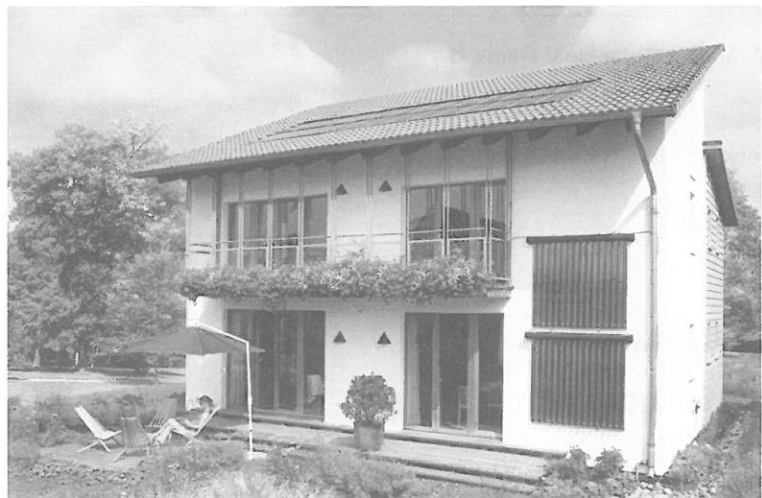
Detached house in Lüdighausen, Germany Photo: Westdeutsche LBS
