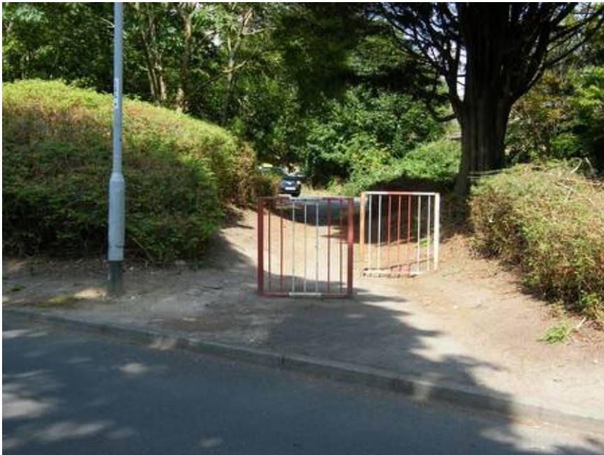
Illustration 1: Exclusionary barriers and missing flush kerb
