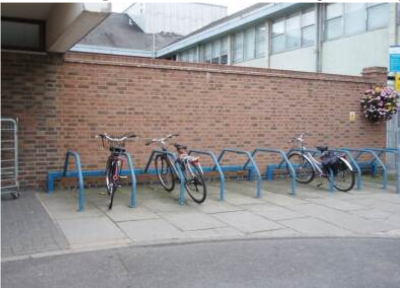
i) Front of Outpatients. Toast racks with inadequate 70cm spacing.
